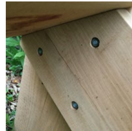
Countersink nuts on inside
